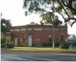
Former Royal Hotel, south and west elevations viewed from the Loddon Valley Highway
