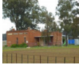
Former Royal Hotel, rear (east)
