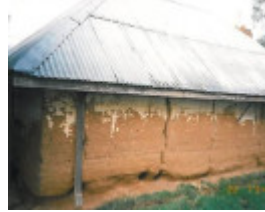
Monmore Vineyard and Buttery Factory, mud brick structure, possibly the 'cooling chamber' of the former dairy
