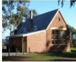
Woodvale Hall, rear (south) and east elevations, note skillion addition at left of picture
