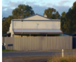
Former Old House at Home Hotel, west elevation, note tall corrugated sheet metal boundary fence
