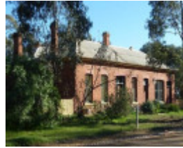
Former Camp Hotel and Store, east elevation
