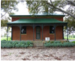
Front (south) elevation of the red brick villa.
