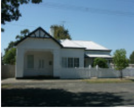
Former Post Office and Residence
