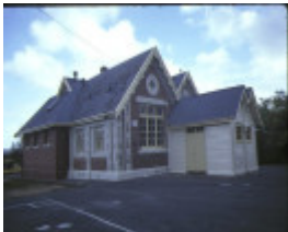
1 primary school number 461 burwood hwy burwood side view sep1984
