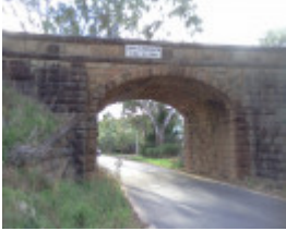
B3602 Blackjack Road Rail bridge
