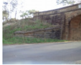
B3602 Blackjack Road Rail Bridge
