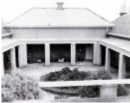
B3974 Piggoreet Homestead Back Courtyard
