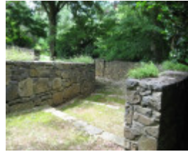
stone walls and steps 2011
