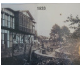
Garden under construction 1933
