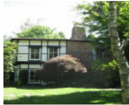
view of house from north 2011
