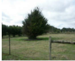
Telstra Substation & Vacant Land
