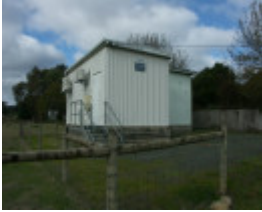
Telstra Substation & Vacant Land
