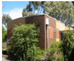
Former Mowbray College toilet block
