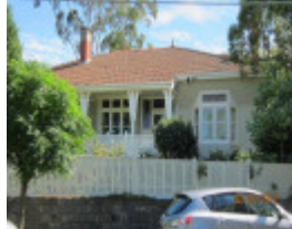
20 Toora Street, Toora Street Precinct
