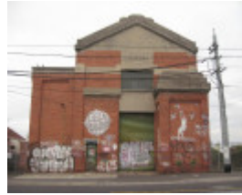
Ascot Vale Substation
