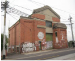
Ascot Vale Substation
