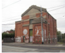
Ascot Vale Substation
