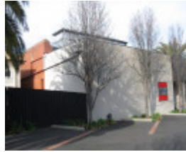
Elsternwick substation rear view
