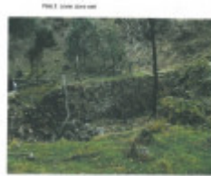
Warby Falls Lower Stone Weir
