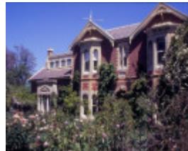
h01188 1 belleville ryrie street geelong front view she project 2004
