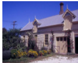
belleville ryrie street geelong stables she project 2004
