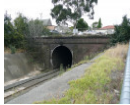
RAILWAY TUNNEL SOHE 2008
