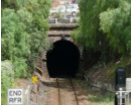
RAILWAY TUNNEL SOHE 2008
