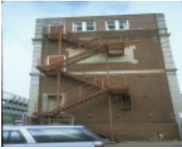
Gordon Technical College Geelong Exterior Staircase August 1995
