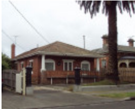
Former Malvern Dairy
