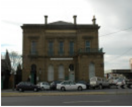
Former Bank - 9-11 Malop Street, Geelong
