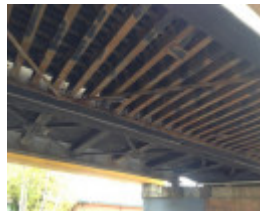
Rail over road bridge Ascot Vale Road
