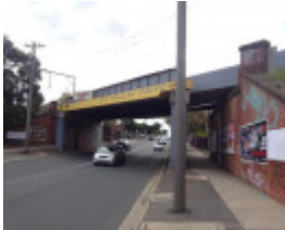
Rail over road bridge Ascot Vale Road
