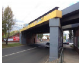
Rail over road bridge Ascot Vale Road
