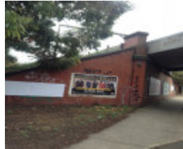
Rail over road bridge Ascot Vale Road
