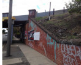
Rail over road bridge Ascot Vale Road
