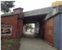
Rail over road bridge Ascot Vale Road
