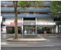
Total House Russell St entrance
