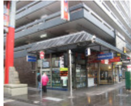
Total House corner shops
