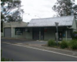
Garage, 849 Heidelberg-Kinglake Road, Hurstbridge, Front
