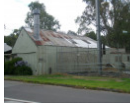
Garage, 849 Heidelberg-Kinglake Road, Hurstbridge, Rear
