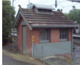
Gardiner switch house
