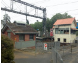
Gardiner switch house (left) and railway signal box (right)
