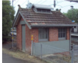
Gardiner switch house
