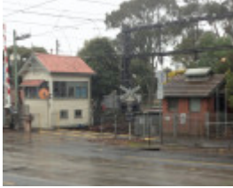
Kooyong railway signal box (left) and switch house (right).
