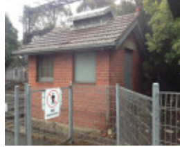
Kooyong switch house.
