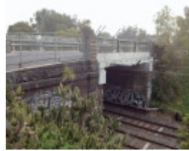
Argo Street Bridge
