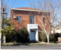
Toorak Telephone Exchange
