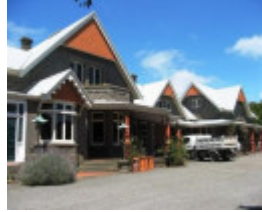
2013 North elevation of house
