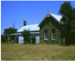
purrumbete camperdown bluestone building
