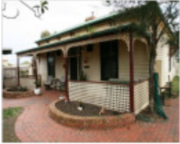
161 Bulmans Road, Melton West
