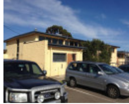
RG Ratcliff Community Centre
