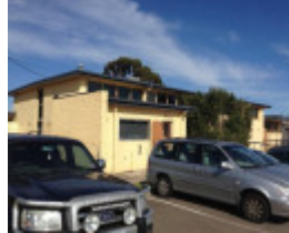
RG Ratcliff Community Centre
