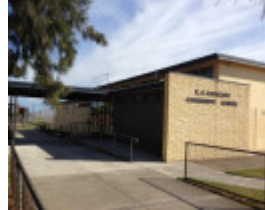
RG Ratcliff Community Centre
