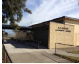
RG Ratcliff Community Centre
