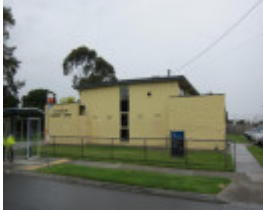
RG Ratcliff Community Centre
