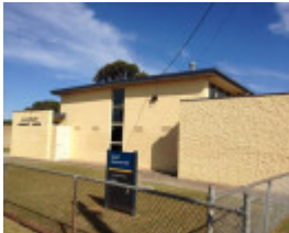
RG Ratcliff Community Centre
