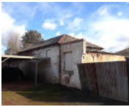
Aberfeldie House Stables
