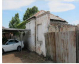
Combermere Street 47 (Aberfeldie house Stables), Aberfeldie (2).JPG
