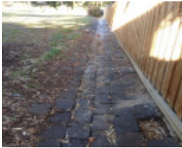
Bluestone drain Brisbane St and Ormond Rd
