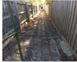
Bluestone drain Brisbane St and Ormond Rd
