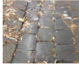
Bluestone drain Brisbane St and Ormond Rd
