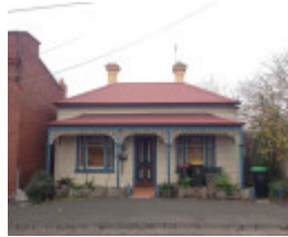
Ascot Vale Fire Station residence (former)
