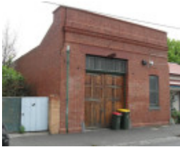
Ascot Vale Fire Station (former)
