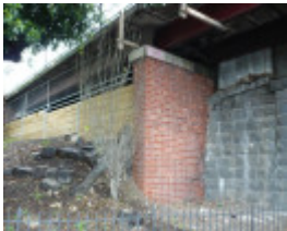
Racecourse Road Bluestone bridge abutment west side
