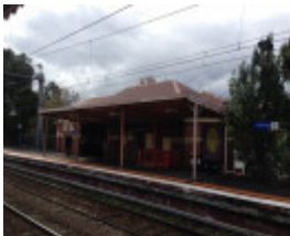
Newmarket Railway Station Up side building
