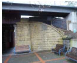
Racecourse Road Railway Bridge abutment east side
