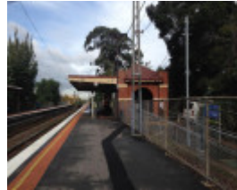
Newmarket Railway Station Down side building
