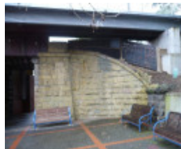
Racecourse Road Railway Bridge abutment east side
