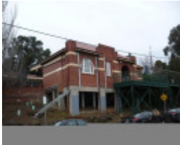
Newmarket Railway Station Up side building (Pin Oak Crescent elevation)
