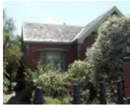
The Crescent 59 a
