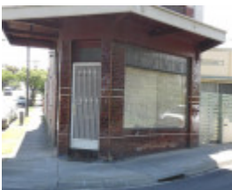
The Crescent 13 c
