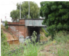
Grice Cr railway bridge.JPG
