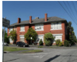
Essendon Primary School No.483 1922 school west elevation
