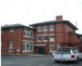
Essendon Primary School No.483 1922 block
