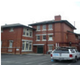
Essendon Primary School No.483 1922 block
