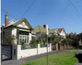
Gardner Street Precinct
