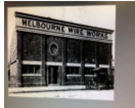
melbourne wire works 85-99 cremorne st c
