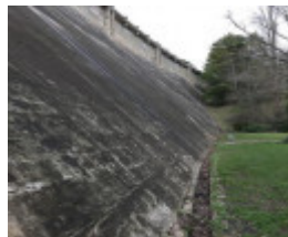
2017, dam wall (2).jpg
