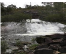
2017, base of spillway.jpg
