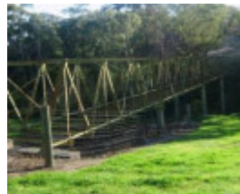
2011, Plenty River pipe bridge.gif
