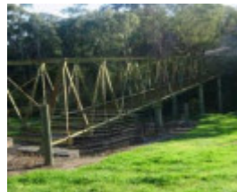
2011, Plenty River pipe bridge.gif
