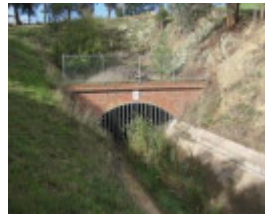
2011, brickwork to tunnel 4.gif
