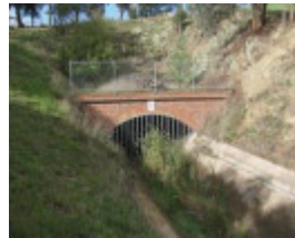
2011, brickwork to tunnel 4.gif
