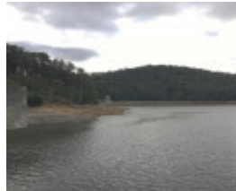
2017 looking north to outlet tower.jpg
