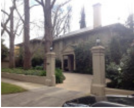
1 Linlithgow Road, Toorak
