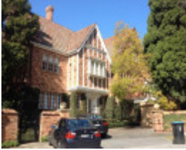
2 Ledbury Court, Toorak
