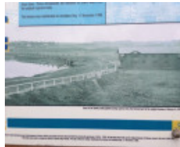
Holmes Road drain outlet 1920 Historic photograph
