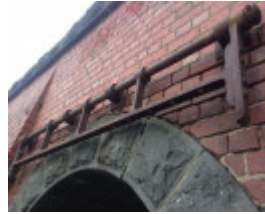
Holmes Road drain outlet
