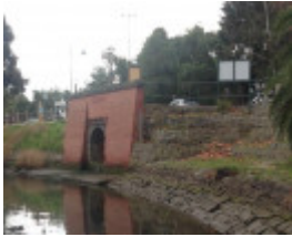
Holmes Road drain outlet
