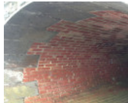
Holmes Road drain outlet
