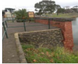
Holmes Road drain outlet
