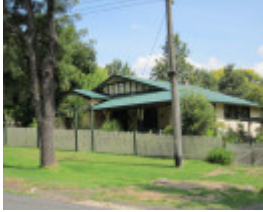
Subject property as seen from Harker Street
