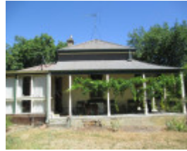
East elevation of residence, with non-original addition at left
