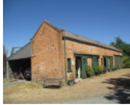
Historic stables building, with lean-to at left.
