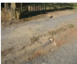
Photo 4 Detail of central stone slab for fastening gates.jpg
