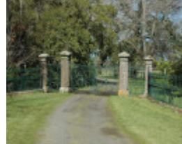
Illustration 3 Gates at Killarney, Dunnstown, 1901 have a similar scale and layout but differ in detail and cast iron pattern. They were designed by George Clegg, architect of Ballarat, who had also designed James Coghlan's home in Ballarat in 1888 and if
