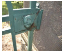
Photo 3 Detail of lock and cast iron handle.jpg
