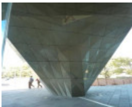
Building pier in main external plaza
