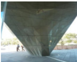
Building pier in main external plaza
