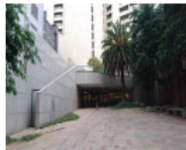
North facade of Shell House from Flinders Lane
