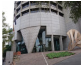
Main external plaza at corner of Spring and Flinders Streets
